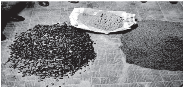
Fig. 3: Mixing of Sand, Cement & Stone
